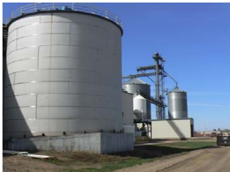
Central MN Ethanol Co-op (CMEC) in Little Falls, Minnesota
